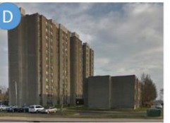
High-Rise / Large Building
