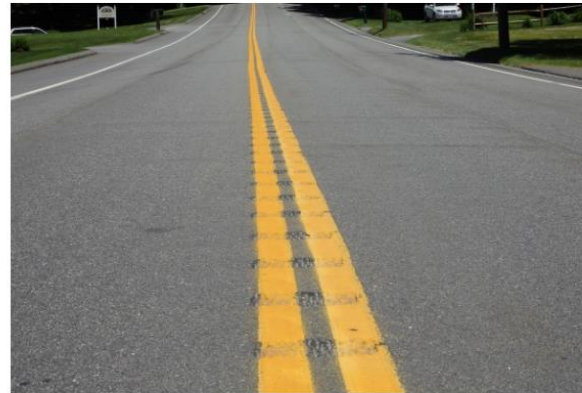
Centerline Rumble Strips (CLRS)
