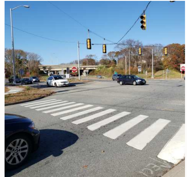
CT-12, US-1 (Long Hill Road) the I-95 (Jewish War Veterans Memorial Highway) Off-Ramp, and Kings Highway
