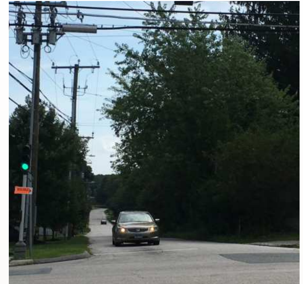
CT-32 (Norwich-New London Turnpike) and Stop and Shop intersection with outdated pedestrian signal on left
