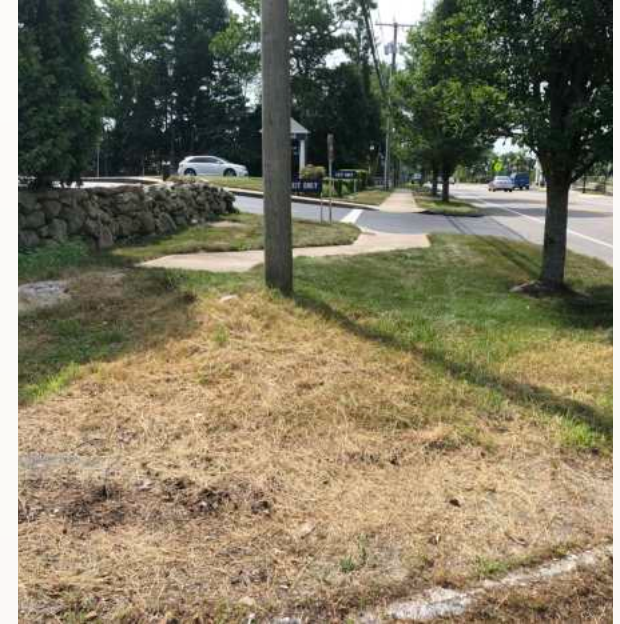
CT-117 (Colonel Ledyard Highway) missing sidewalks
