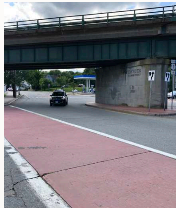
US-1 (West Broad Street) Railroad Abutment
