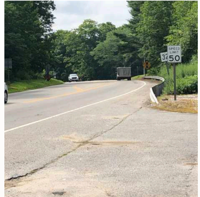
CT-32 (Franklin Turnpike) near CT-87 (Norwich-Lebanon Road)
