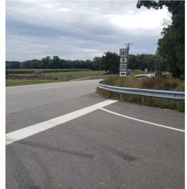
CT-201 (Glasgo Road) and CT-165 (Shetucket Turnpike)
