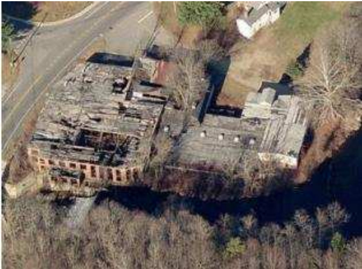
The abandoned Norton Paper Mill building and dam in 2015. Source: connecticutmills.org / Bing
