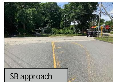
Route 161 (Pennsylvania Avenue) and State Road and Lincoln Street is an unsignalized four way intersection with Lincoln Street on the east side of Route 161 and State Road to the west. Both State Road and Lincoln Street are Stop controlled with a one lane approach. Route 161 is uncontrolled and has one approach and departure lane in each direction. There is a crosswalk across the southern leg of Route 161.
