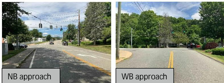
Route 161 (Flanders Road) and Roxbury Road is a signalized T-intersection with Roxbury Road forming the stem of the Tee on the west side of Route 161. All legs of the intersection have one undesignated approach lane and one departure lane. The traffic signal is uncoordinated and operates on a single controller with the signal at the intersection of Route 161, East Pattagansett Road and Chapman Farms Road.
