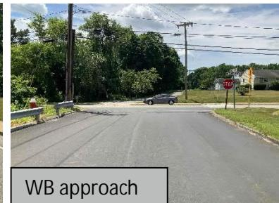
Route 161 (Pennsylvania Avenue) and Oswegatchie Hills Road is an unsignalized T-intersection and Oswegatchie Hills Road is stop controlled with a single approach lane. Route 161 is uncontrolled and has one approach and departure lane in each direction. There is a crosswalk across the western leg of Route 161.
