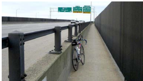
Figure 2.12. Narrow bike and pedestrian conditions on Gold Star Memorial Bridge
