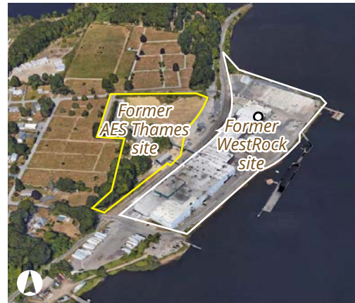
Figure 3.19. Location of former AES Thames and WestRock paperboard plant (Google Earth)
