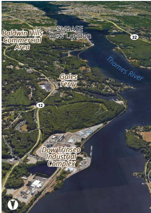
Figure 2.47. The Dow Trinseo industrial complex with SUBASE New London to the south in the background (Google Earth)
