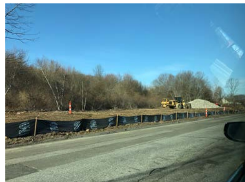
Figure 2.39. Crystal Lake Road improvements under construction
