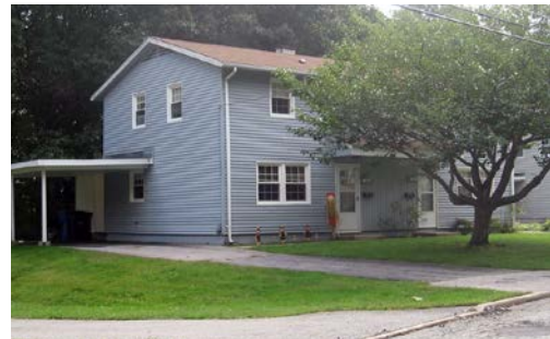
Figure 3.30. Navy housing at Nautilus Park II (Balfour Beatty Communities)
