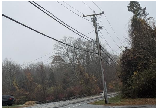
Sight line is blocked by vegetation south of the fire station driveway.
