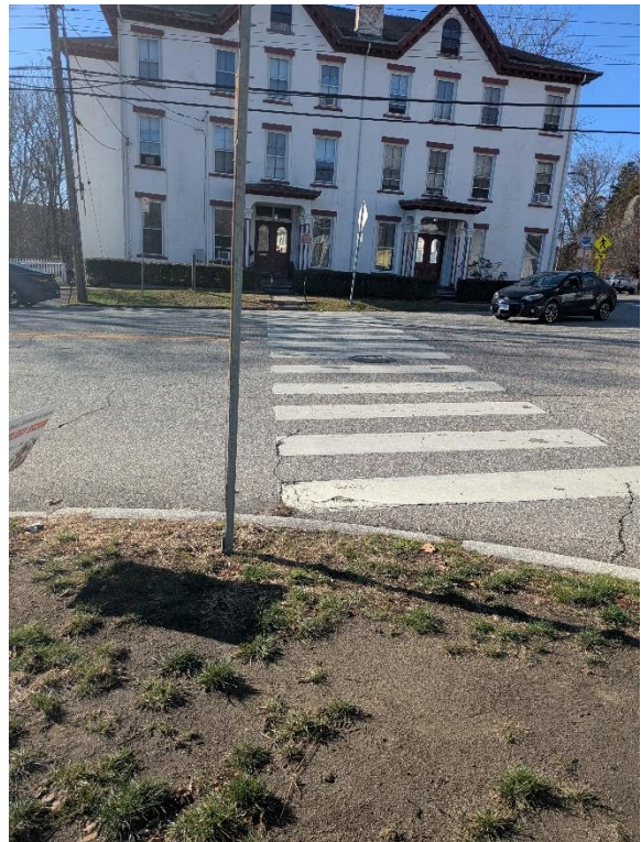
Existing crosswalk across the southern leg of the intersection.
