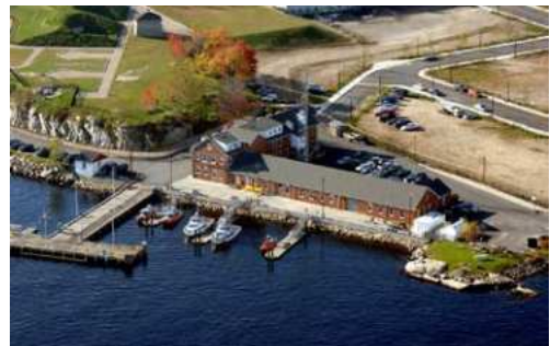
Figure 2.67. USCG Station New London (USCG)
