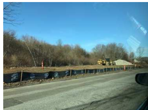
Figure 2.39. Crystal Lake Road improvements under construction
